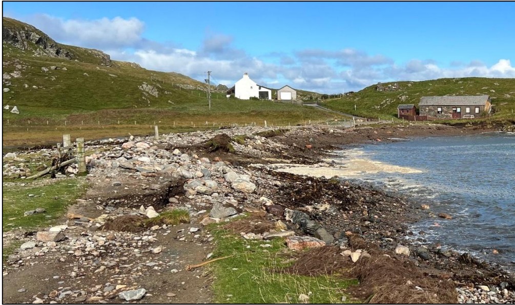
v ii. Coastal erosion at Bousta beach
