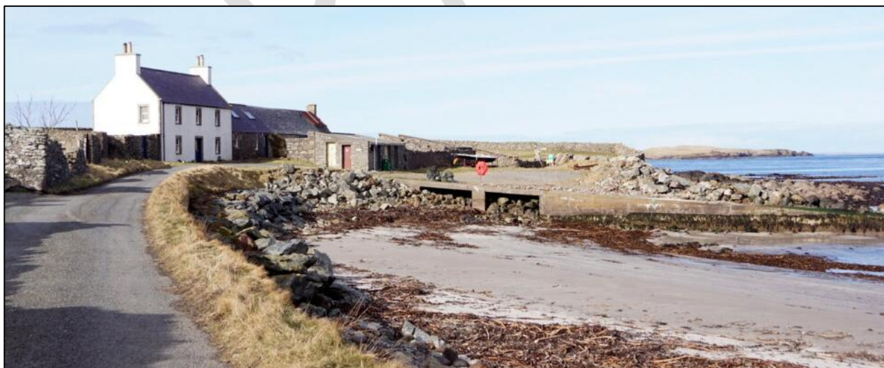
North House and the Melby pier site
